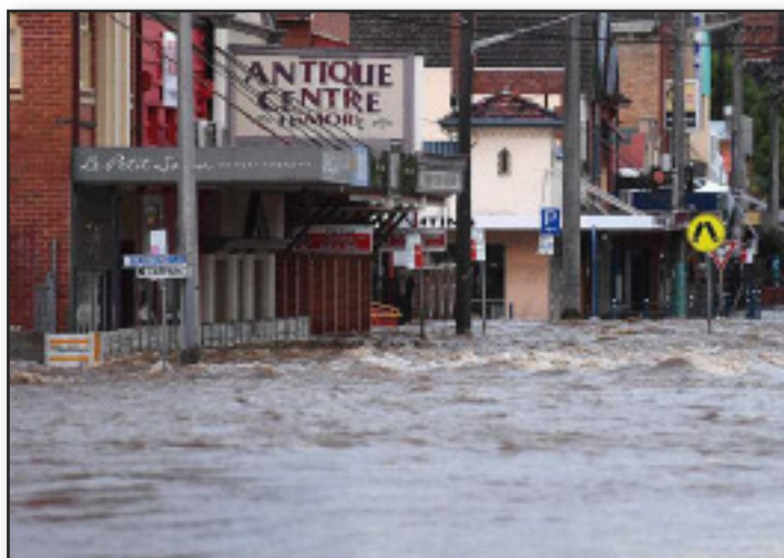
The flooded town of Lismore Northern NSW.
