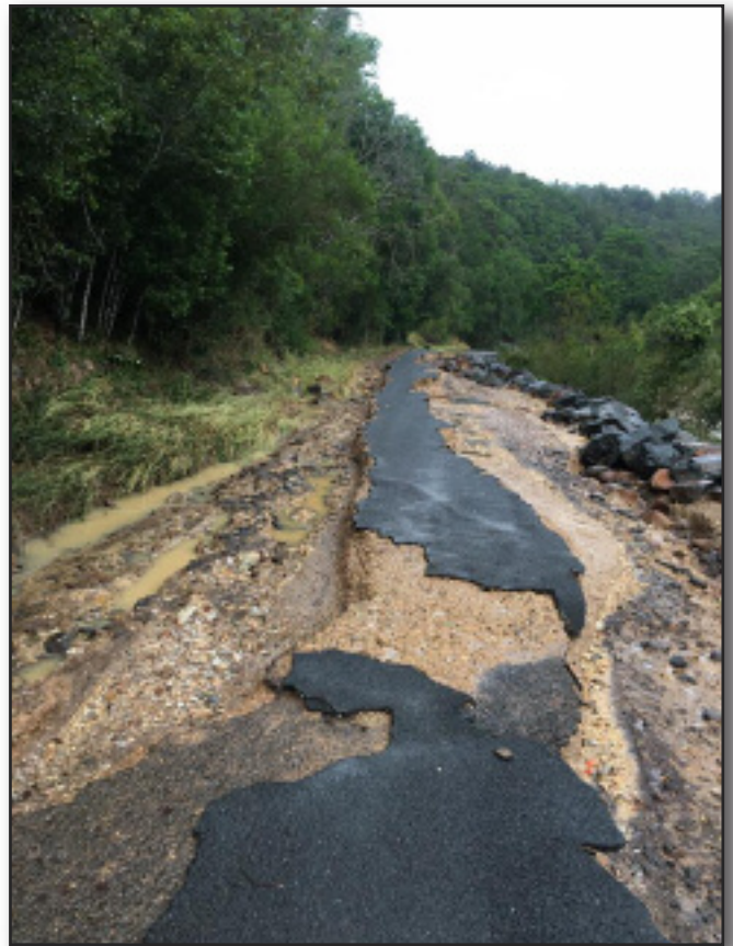
Only road in and out destroyed at Burrill Creek.
